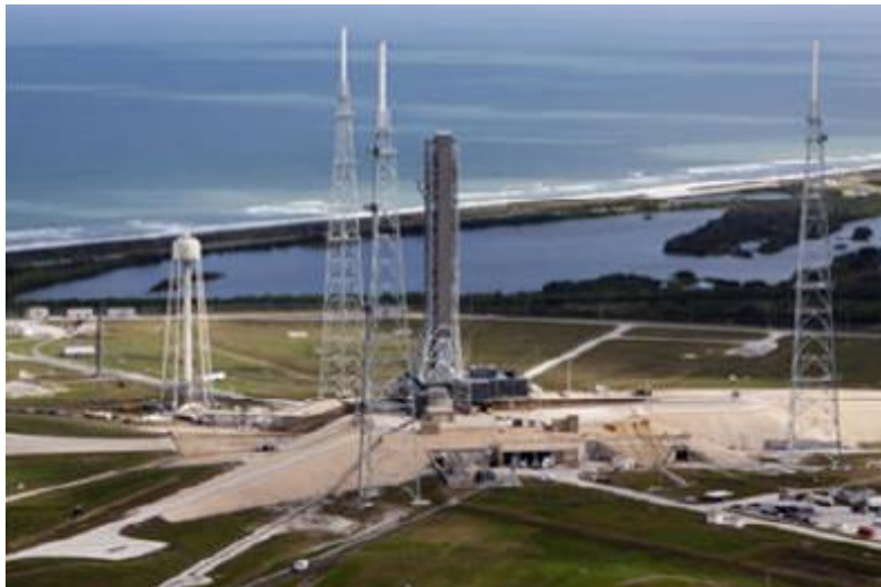
Figure 7-12. Launch Complex 39B (LC-39B)
