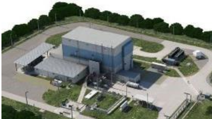
Figure 7-4. Multi Payload Processing Facility (MPPF)
